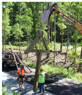
Constructing the kiosk at Morse Road.
