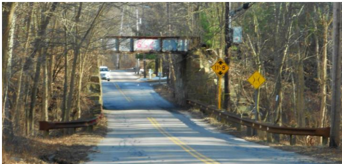
The Grove Street Bridge on Phase 2 of the trail in Framingham.
