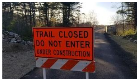
The bridge construction area is closed until completed.
