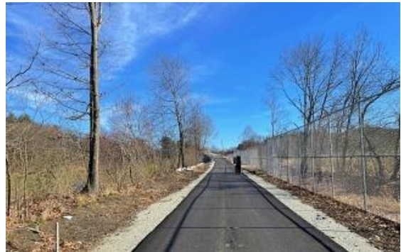
Access to the Rte. 2 bridge viewed from Acton, with the State Police Barn fencing on the right.
