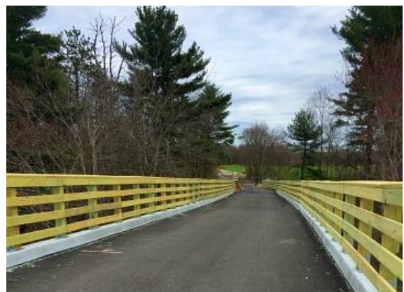
New railings on the bridge access ramp from Concord.
