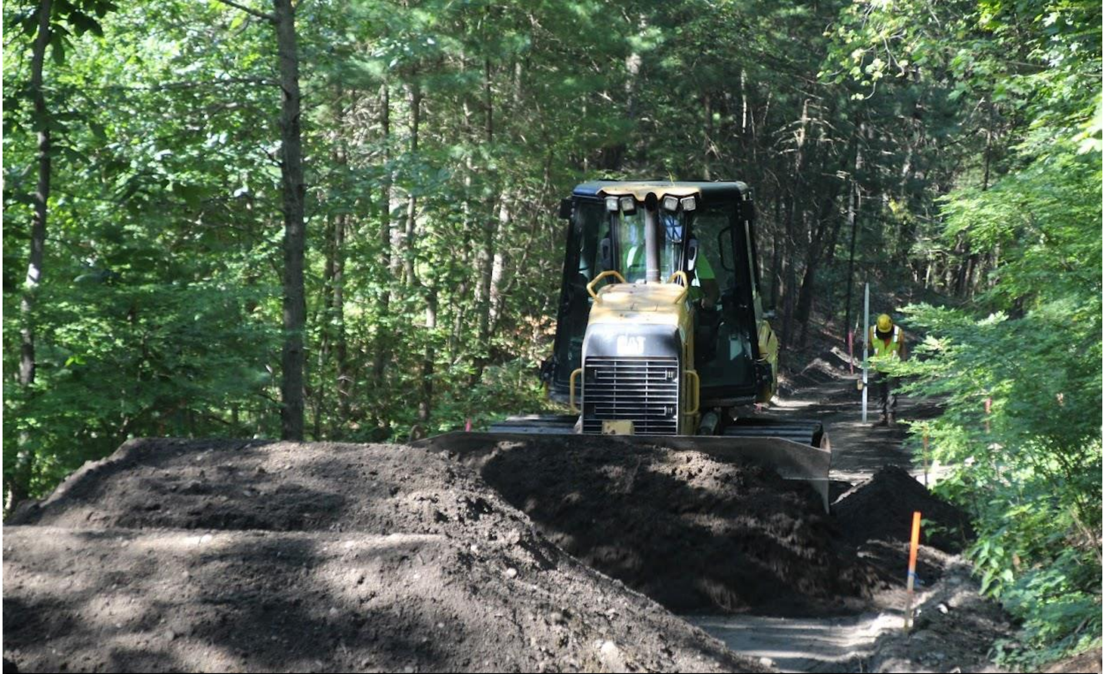
August 7, 2023: Leveling and grading of subsurface material at Old Lancaster Rd.
