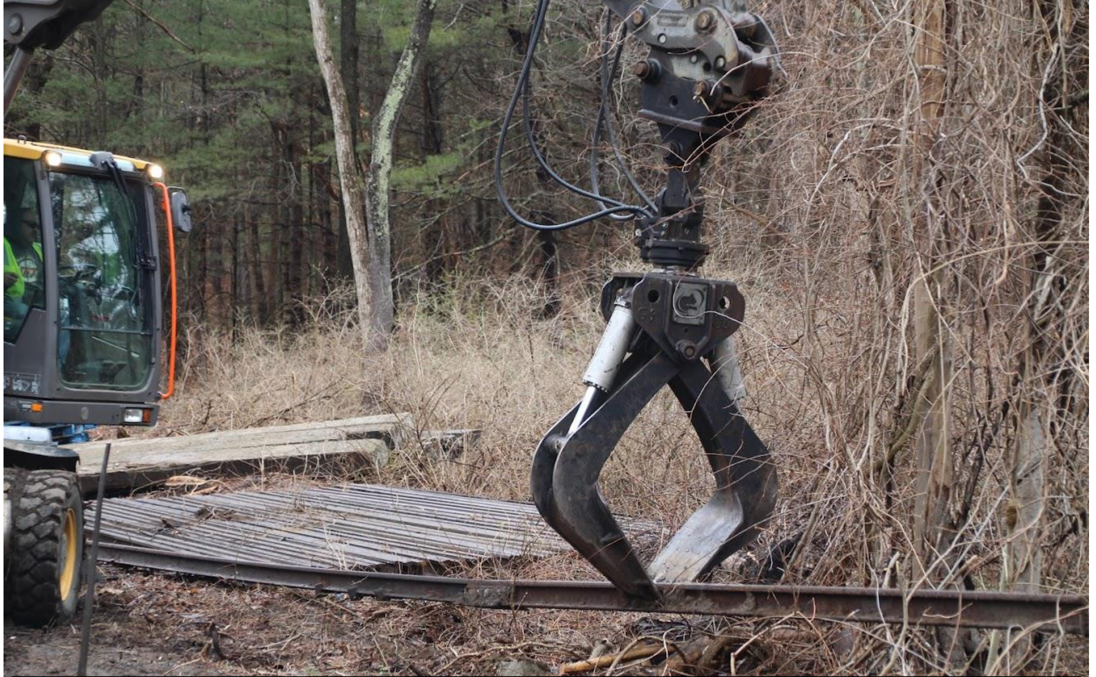
March 28, 2023, Specialized equipment removing rails for salvage or reuse, Ti Sales.
