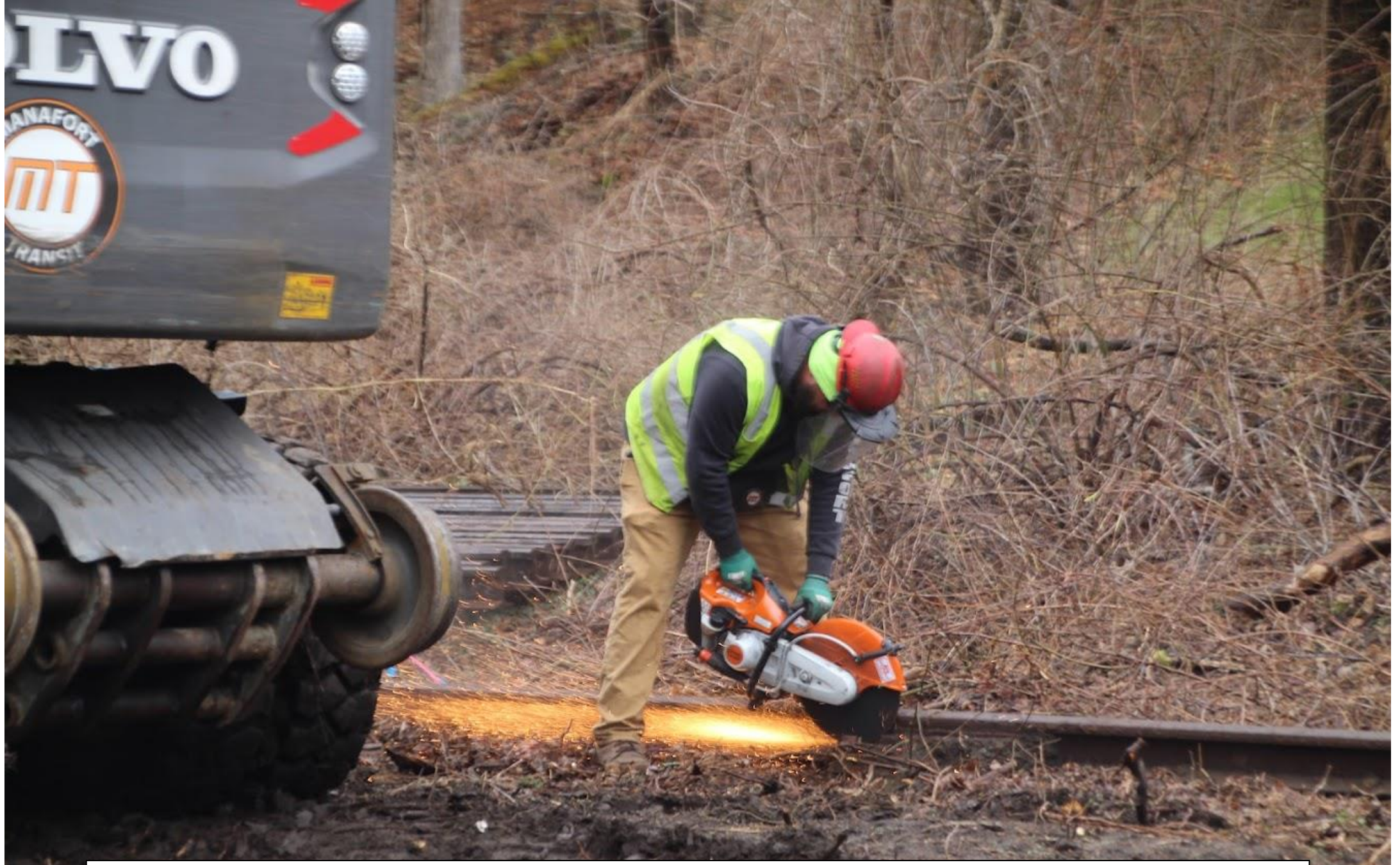
March 28, 2023, Steel cutting saw removing bolts to disassemble rails.
