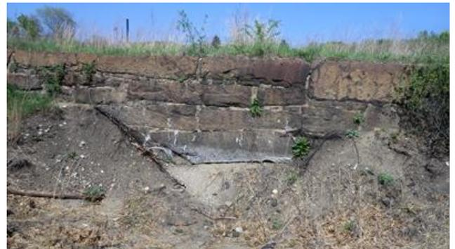
A portion of the wall further down the track was recently excavated revealing the entire wall down to its foundation.
