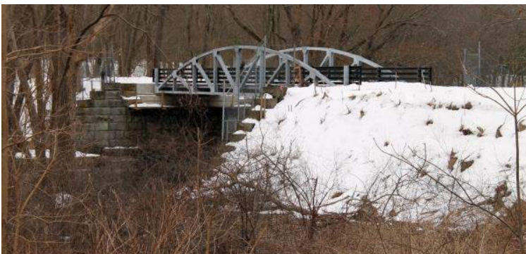
The bridge over the Assabet River in West Concord was installed last fall. Photo was taken from the back of Westgate Park car wash site.
