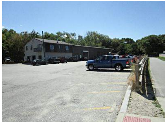
Grist Mill Apartments At Beaver Brook, a new apartment building project, is being planned for this area near Cushing Place in Chelmsford Center. (View is from near the kiosk.) The project will include reconstruction of the BFRT parking lot with associated landscaping and lighting. The developers will also landscape and maintain the section of trail in front of the retaining wall with the Art Walk murals that separates the trail from Ginger Ale Plaza.
