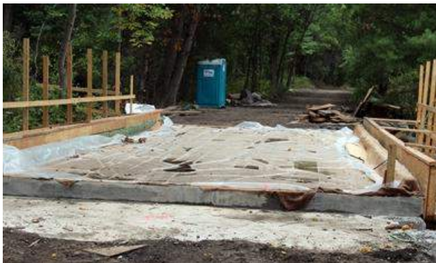
One of six small historic bridges being rebuilt over brooks and streams in Acton. The top course of original stones is being reset onto the new deck..
