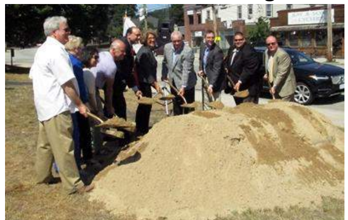
Tom Kelleher, President of the Assabet River Rail Trail (left) with local and state government representatives at the groundbreaking in Maynard. This new section of the ARRT is 3.5 miles, running from the South Acton MBTA station, through downtown Maynard, ending at the Stow town line.
