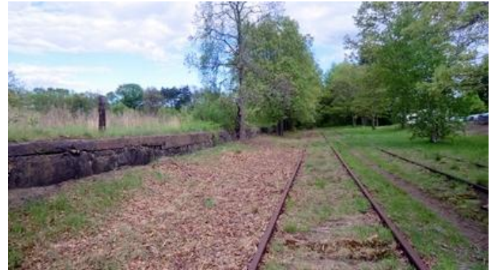
This historic retaining wall next to the tracks in West Concord was likely built around 1900 when the nearby yard trackage was expanded.
